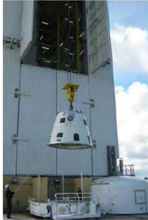
Figure 6.2.3.2.1e – Hoisting and integration of the 1/2 interstage
